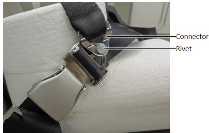
Figure 21. Connector Attached to Rivet
